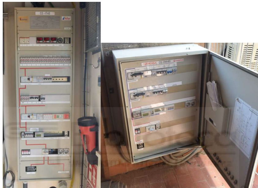
Figura 11 CGBT Trifásico 400V Interior y CGBT Monofásico 230 Exterior
