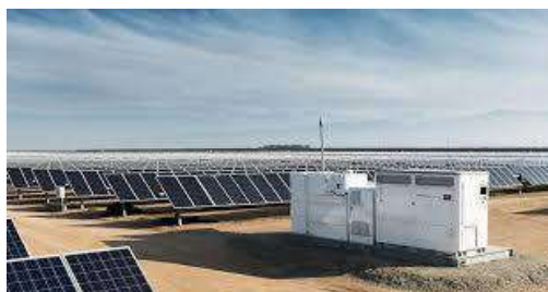
Figura 43: Inversor central
