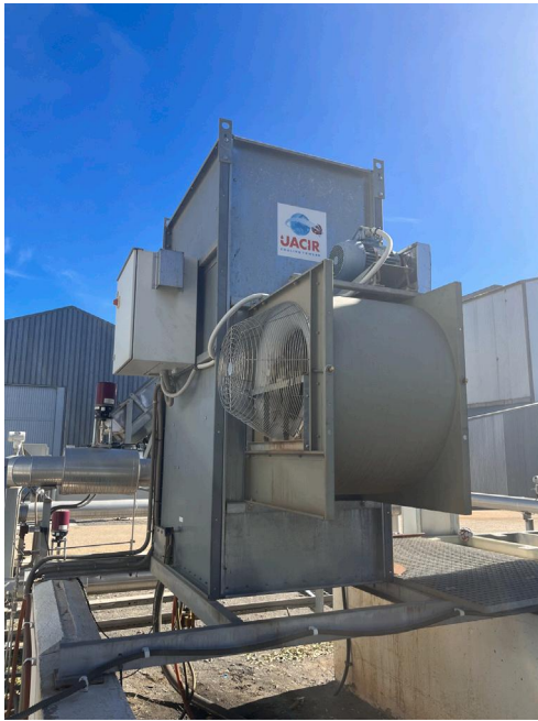
(b) Forced mechanical draft wet cooling tower.
