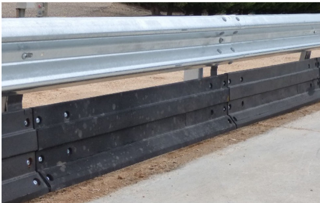
Figure 16. Installation out of the paved surface.
