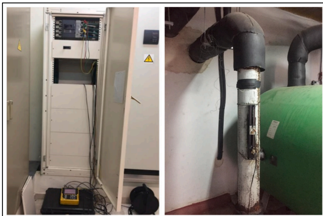
Fig. 10. Sensors installed in the facility. Power meter (left) and flow meter (right).
