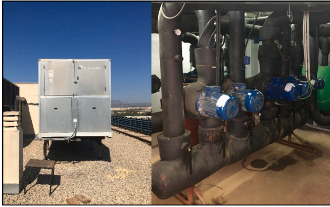
Fig. 4. Heat pump (left) and circulation pumps (right) of the facility.
