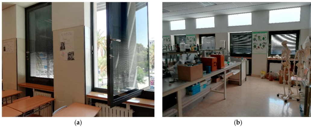
Figure 11. (a) Hinged window with a sophisticated system of venetian blinds incorporated in between the two glass sheets of the window are expensive to repair. (b) Hinged windows reduce the amount of useful space in the room. They are not functional.
