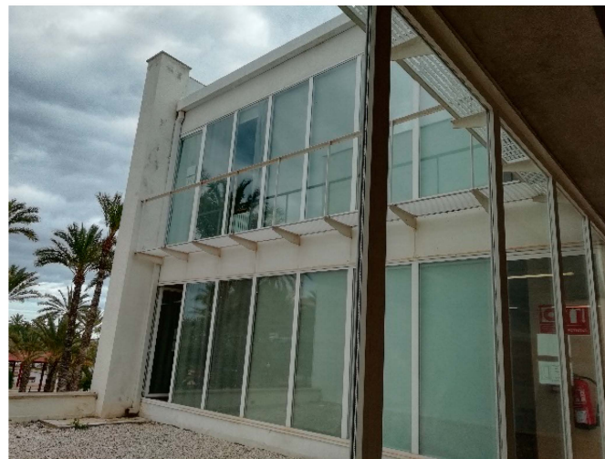
Figure 12. “Walk-out windows” seen from the outside.
