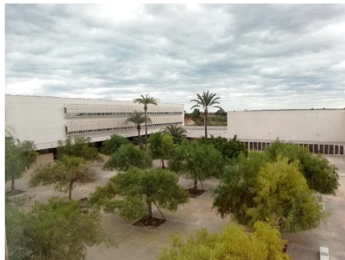
Figure 16. Fixed blades and trellis, as seen in many modern school buildings, may have an aesthetic function from the outside but are not visually comfortable for users from the inside (see Figures 5 and 15).
