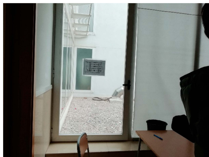
Figure 13. Hinged, “walk out” window seen from inside of the classroom. The difficulties of opening these windows lead to tolerating higher temperature in the rooms.
