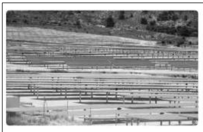
Figure 3. Solar panels installation in Alicante.
