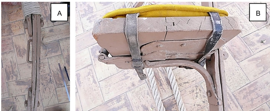
Fig. 14 A Forged steel plates fixed with screws and rope added. B Forged steel support situated under the lateral ledges
