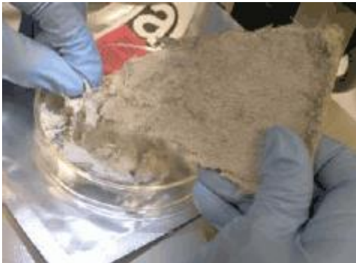
Figura 3. 4. Material friable. Panel.[7]
