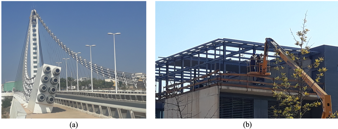
Figure 2.1: Vertical structures require inspection and maintenance tasks which are dangerous for human operators due to several risks, including falling from considerable heights. Examples of structures requiring operators working at heights: (a) Bimillenary's Hanger Bridge of Elche, (b) expansion works at the Quorum III building of the Miguel Hernández University.
