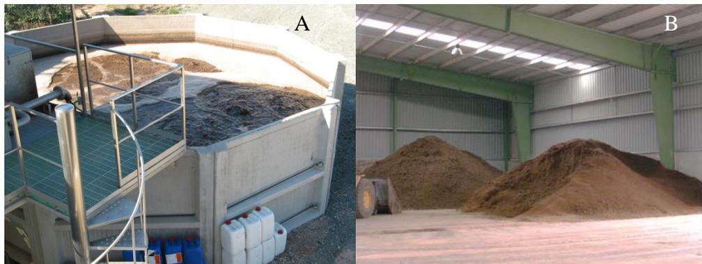
**Figure 6** – Pig waste storage facilities: A – slurry storage; B – solid fraction storage.
