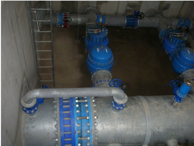
Fig. 6. Detailed view of the inside of a representative manhole.
