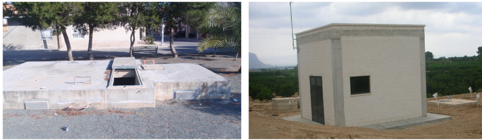
Fig. 5. Two examples of typical underground (left) or booth (right) water management facilities.
