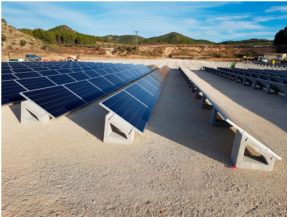
Figure 13. Photovoltaic installation. Figure 13. Photovoltaic installation.
