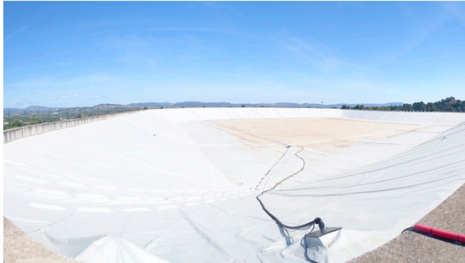
Figure 9: Waterproof sheet in reservoir to reduce evaporation. Source: Own.
