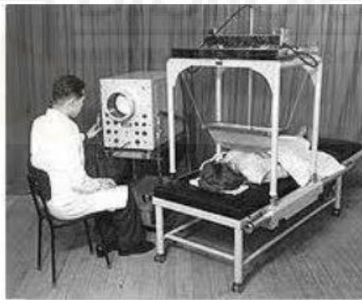
**Figure 7: The water-bag B-mode scanning system, the SSD-1, from Aloka in 1960**
